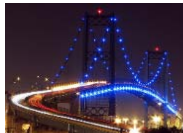
Vincent Thomas Bridge, San Pedro (near Long Beach), CA (each blue light is a string of 7 blue LEDs powered by NCP1216)
