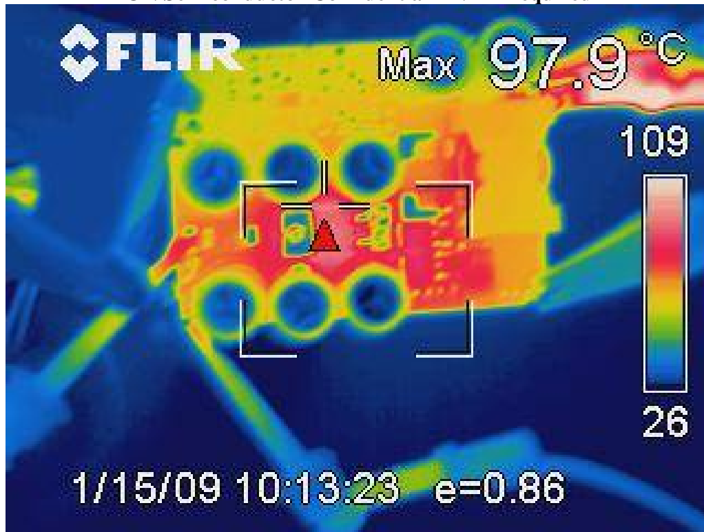
Figure 18: Thermal Image of PCB at 12V 8.3A Load with a 25C ambient
